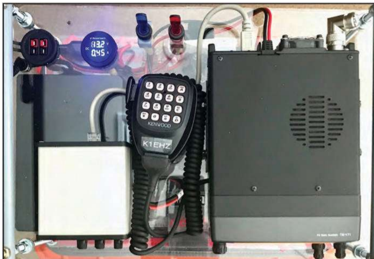
Photo B. Equipment placement on the upper level.
